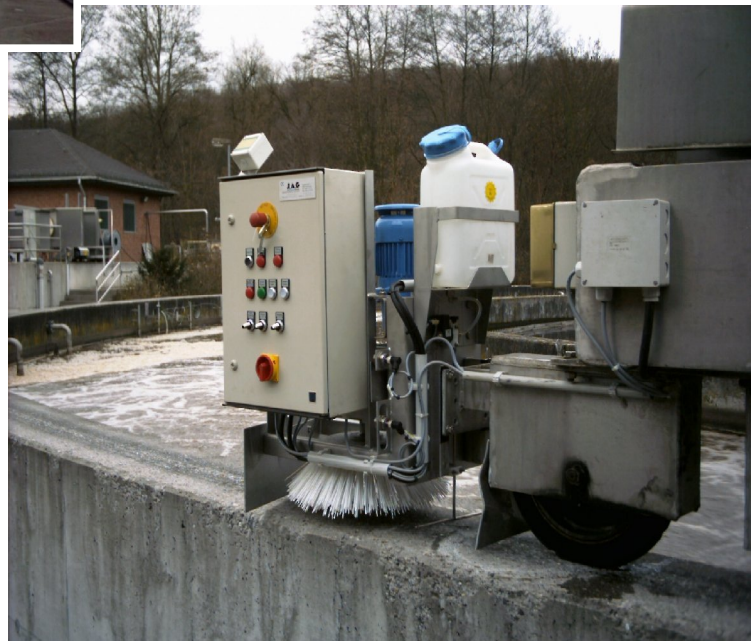
Automatic device with integrated control
