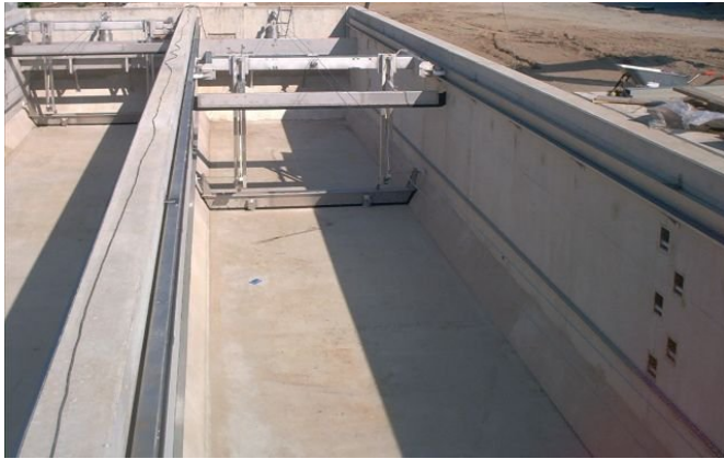
Cable pull scrapers in a double basin
